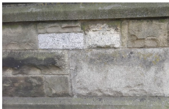
Figure 8. One of the stone panels. H of P- Houses of Parliament. St.P – St Pauls, London. S'M – St Martins le Grand, York, M – Leeds City Museum
