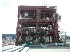
Figure 3. Damaged Buildind by the 2011GEJET
